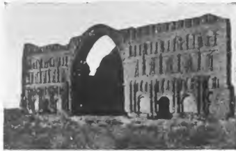
Fig. 508.—Ruins of the Palace of Ctesiphon. Persia. (Dieulafoy.)
